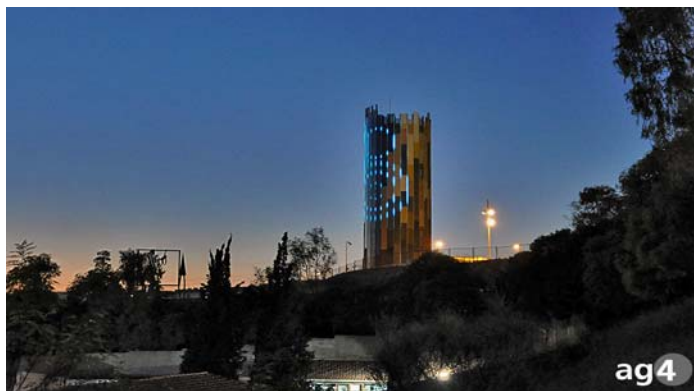
Foto 3: Balance Tower, 2009, © ag4 mediatecture company.
