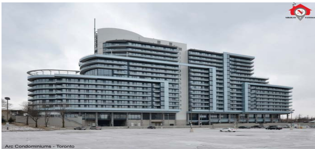
Fig. 15. Arc Condominiums Building – Toronto Source: Toronto Real Estate Guide, The Nikolay & Tatiana Real Estate Team. Sutton Group- Admiral Realty Brokerage
