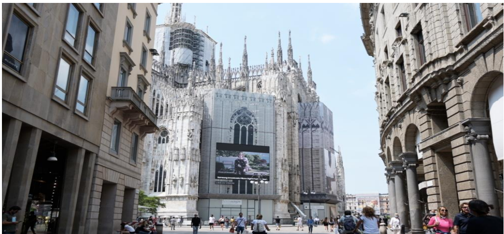
Fig. 15. Super-sized digital signage from Samsung Electronics installed at the Duomo Cathedral in Milan, Italy-January 2021.
