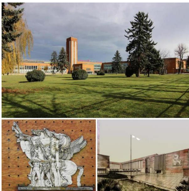
Fig. 4. Administrative complex and club designed by architect Octav Doicescu, IAR-Braşov, 7 Turnului Street, Braşov 1937-1938
