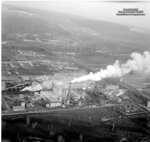
Fig. 10. Suceava Industrial Zone, with the Pulp a Paper Mill in operation – view from the plane.
