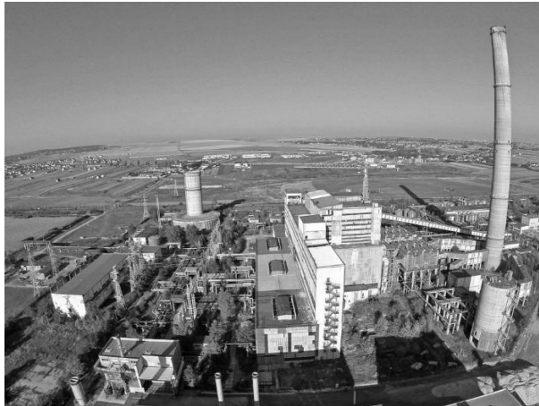
Fig. 11. The the Artificial Fibres Enterprise with the IFA Tower on the right
