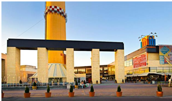
Fig. 12. The Iulius Mall Suceava shopping complex with the IFA Tower base
