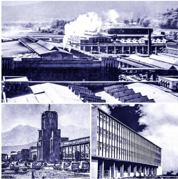
Fig. 2. IAR – Romanian Aviation Industry, which became Stegul Roşu Factory, production hall and administrative building, Braşov, 1927
