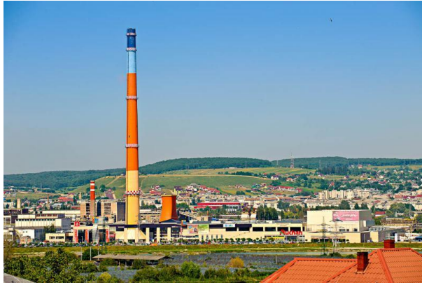
Fig. 12. The Iulius Mall Suceava shopping complex with the IFA Tower
