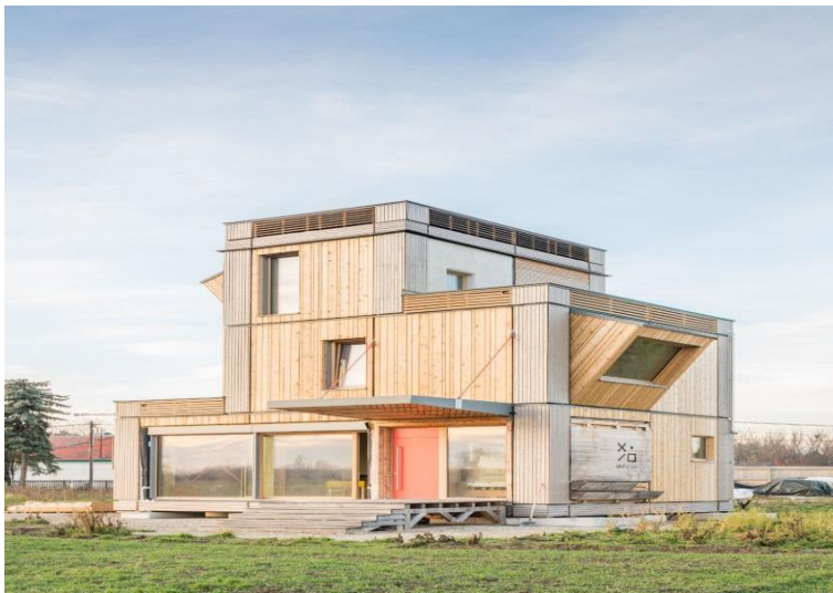
Fig. 7. The modular construction system Vivihouse project
