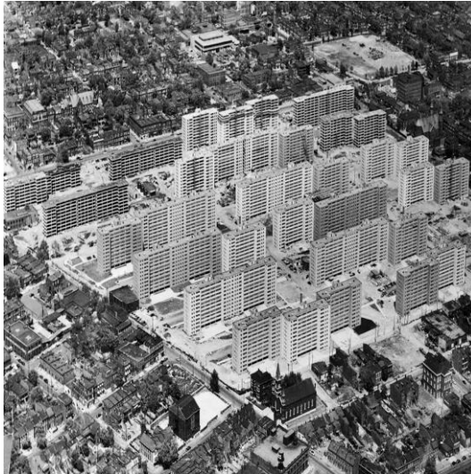
Fig. 21. Pruitt-Igoe Social housing in St.Louis,after completion in 1956.
