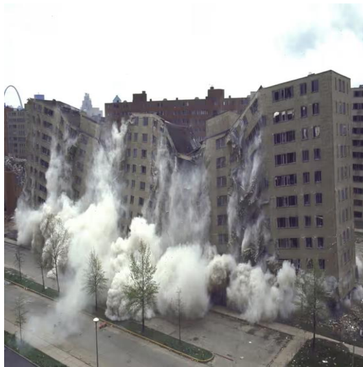
Fig. 22. Second phase of demolition of Pruitt-Igoe , April 1972. Photo credits Lee Balterman/Time & Life Pictures/Getty Images
