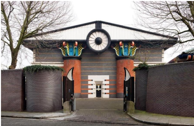
Fig. 5. Architect John Outram - Isle of Dogs Storm Water Pumping Station, London
