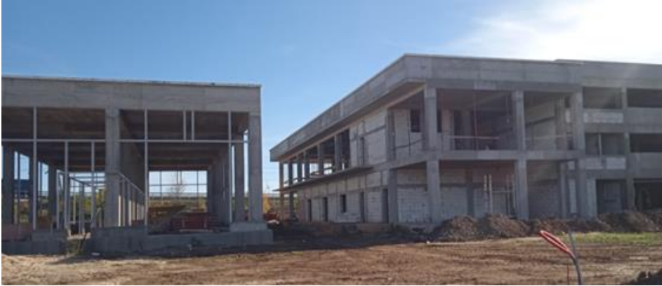
Fig. 8. During execution; Source: archive of the Alexandria city hall
