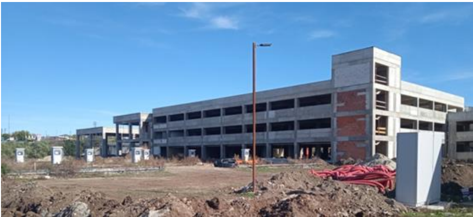
Fig. 9. During execution; Source: archive of the Alexandria city hall
