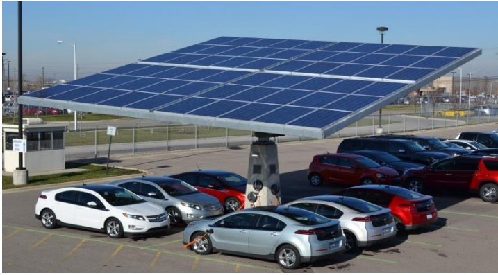
Fig.2 A photovoltaic parking with EV chargers included
