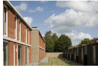
Fig. 8. 30 Senior Housing / Bastiaan Jongerius Architecten Source: https://www.archdaily.com/410233/30-senior-housing-bastiaan-jongerius-architecten?ad_source=search&ad_medium=search_result_all
